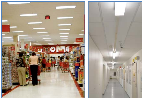
Figure 2. Luminaires that are within the normal field of view feature diffusers, resulting in low radiance (left photo: wiki public domain).
