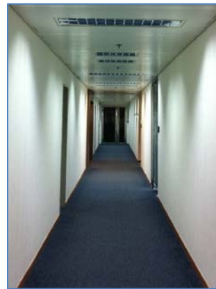
Figure 3. In this example, the lamps are not covered but are shielded by reflectors so that they are only in the field of view when one looks up (photo by Hsiaoheitoo, CC BY-SA 3.0)
